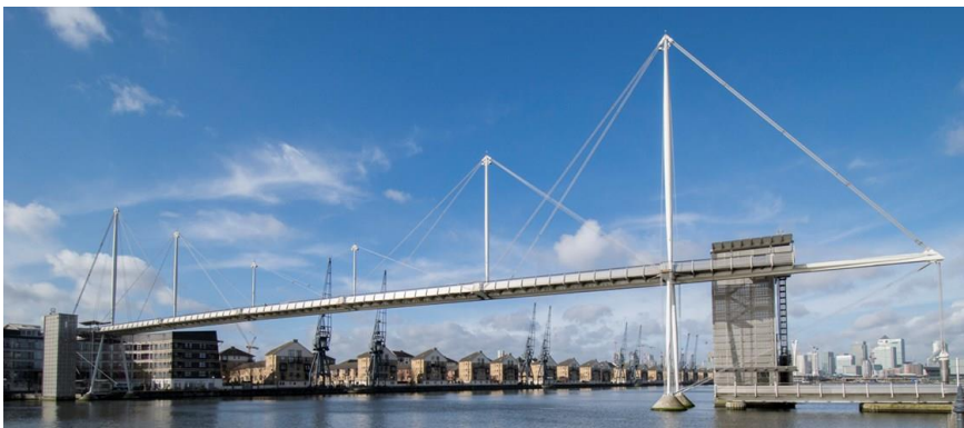
Рис. 5. Royal Victoria dock bridge
